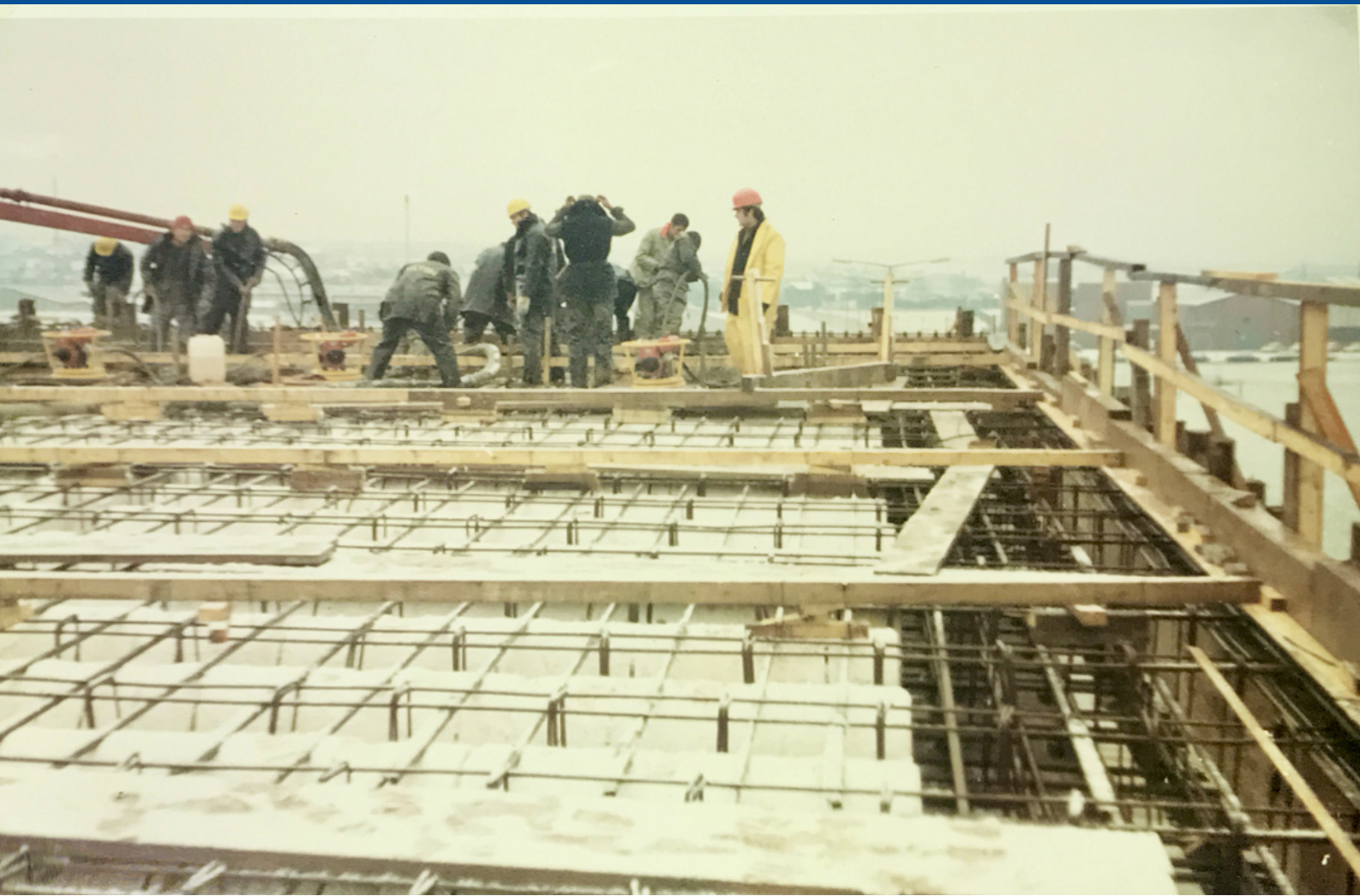
Construction of Gillibrands Bridge after snowstorm, February, 1970.
